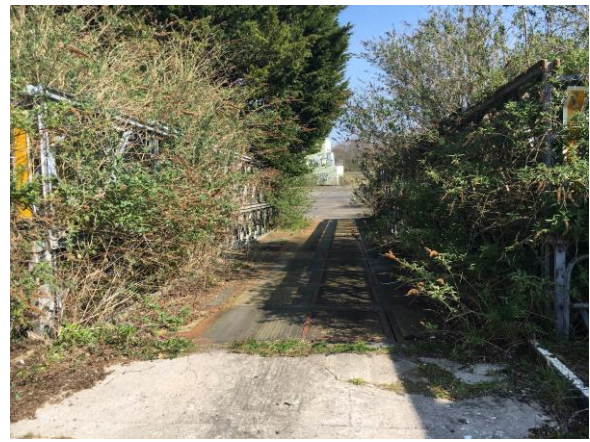
Bridge crossing the Mill Leat between the south and north sites
